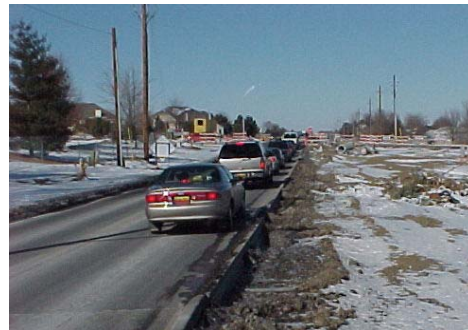
132 nd Street looking north at the Blondo Street intersection.
