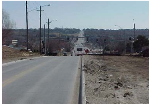
Blondo Street looking east at the 123 rd Street intersection
