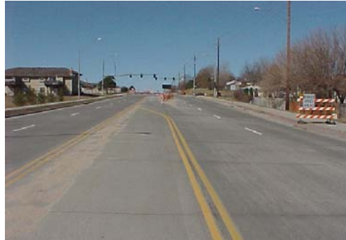
Looking west on Blondo Street at 123 rd Street
